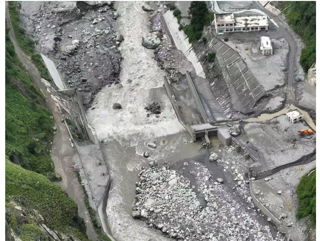
Destroyed hydropower plant
